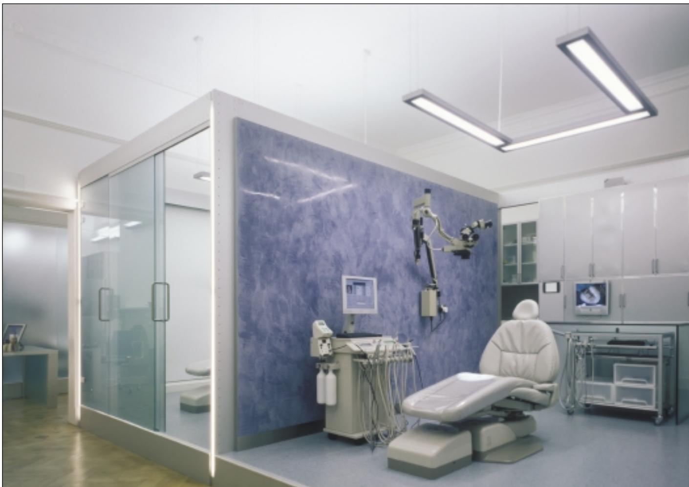
**Figure 4 (above):** Operatories are built into aluminium 'pods' supported on raised floors
